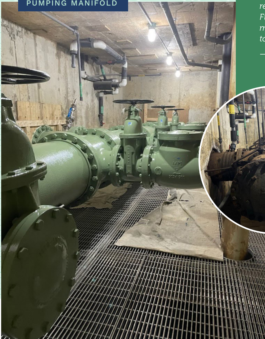
NEW RAW WATER PUMPING MANIFOLD
